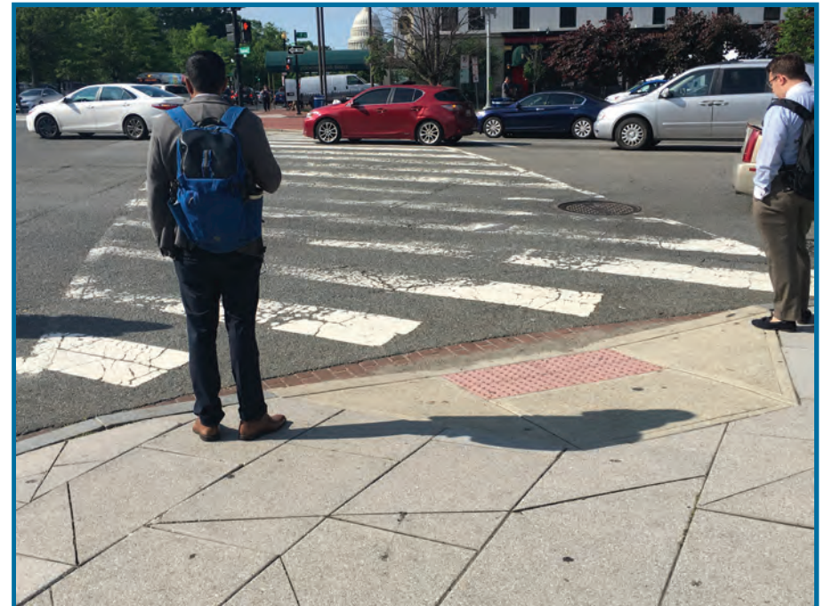
Crosswalk needing restriping at N Capitol Street and Massachusetts Avenue.
