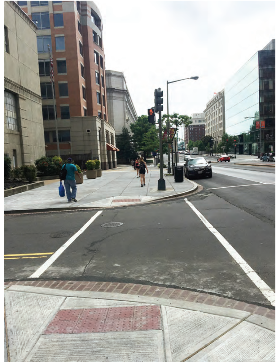
Wheelchair ramps are in good condition crossing G Place NE.
