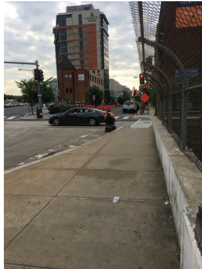
While the sidewalk is wide, the people in wheelchairs use the street, because the curb ramps are not ADA compliant.
