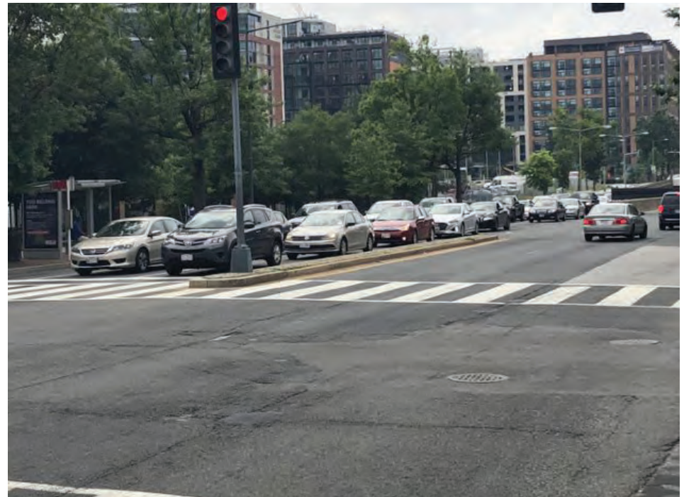
Median nose extends into the crosswalk, creating a trip hazard for visually impaired or distracted pedestrians.
